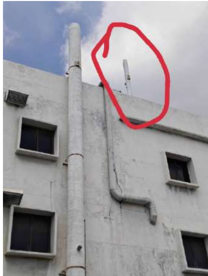
Chimney 6 (R&D lab)
